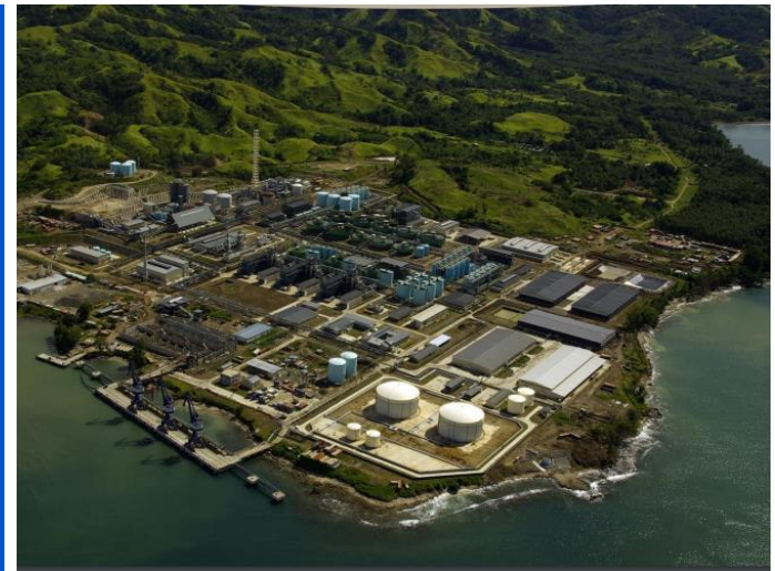
Basamuk Processing Plant
